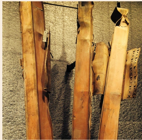
Deformed steel beams after a fire.
