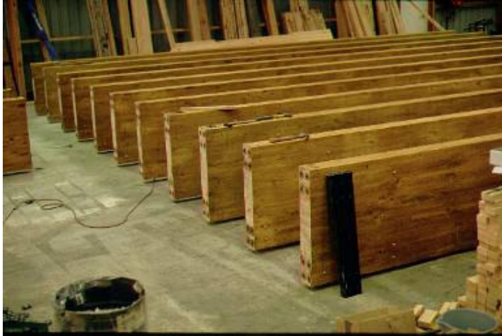
Figure 3.4: Prefabricating laminated beams
